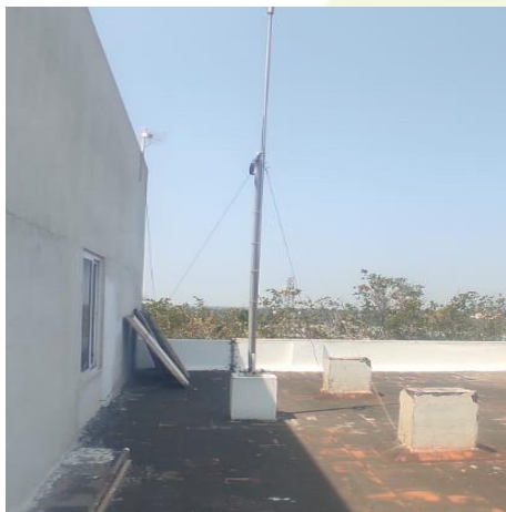
Lightning Arrestor
